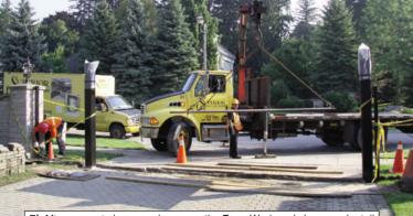
5) After concrete has cured, remove the Form Work and clean up. Install the Control Panels, Junction Boxes, and Photo-Cells. Install the PVC Conduit for Controls, Safety Equipment Lights, and spares for future use.
