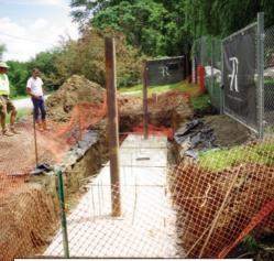
2) Install heavy duty Steel Posts by bolting to the Concrete Foundation Base to support the Heavy Gates.
