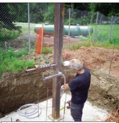
3) Weld Steel Hinge Extensions, Motor Brackets, Photo-Cell and Light Extension Brackets. Install PVC Conduit for Power, Controls, Safety Equipment and Communication.
