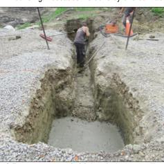
1) Excavate 1200mm [4 ft.] deep for both gate pillars and across the driveway. Pour 200mm [3" ] Concrete Foundation Base. Install heavy duty Steel Posts by bolting to the Concrete Foundation base to support the Stone Pillars.
