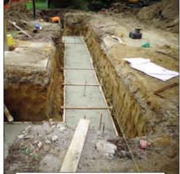
1) Excavate 1200mm [4 ft.] deep for both gate posts and across the driveway. Pour 200mm [8" ] Concrete Foundation Base
